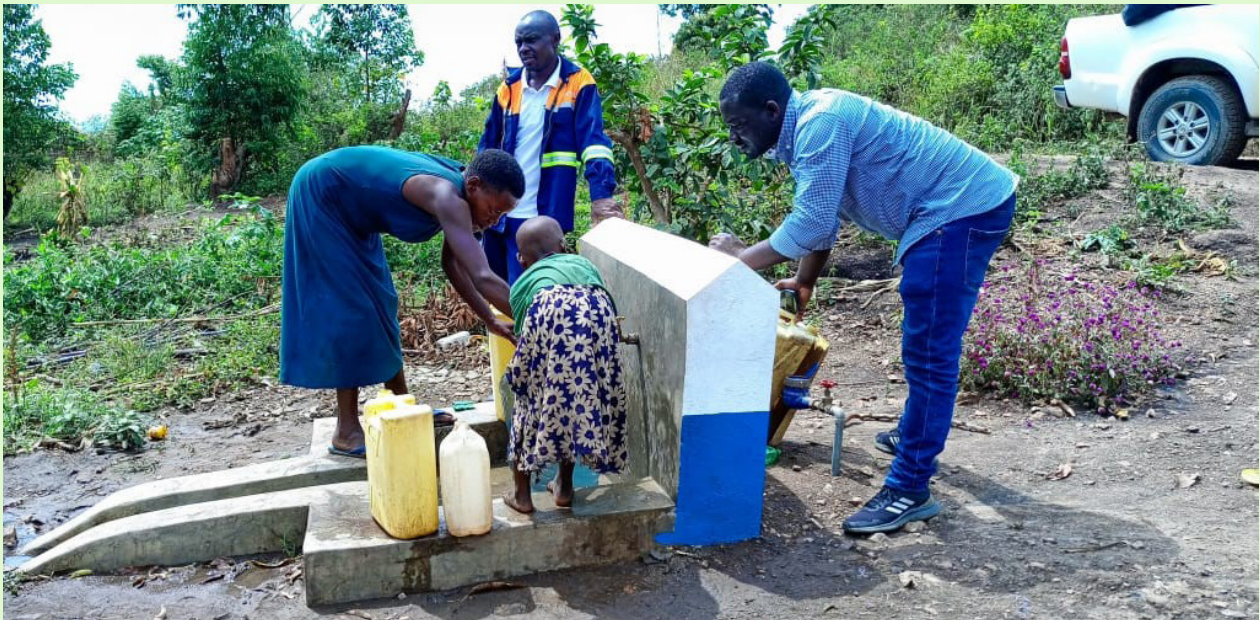
Community members in Ntara sub county collecting water from the recently completed Rwentuha-Ntara water project that was implemented by Jese in 2024
