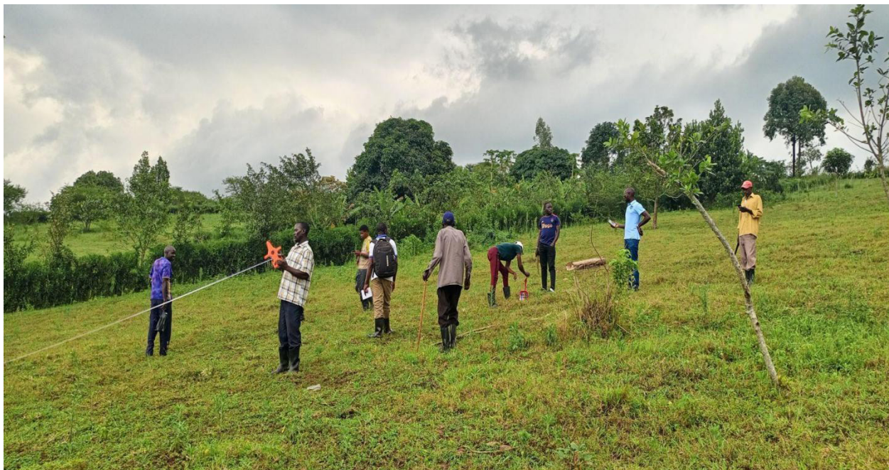
Community members of Rwenjaza Sub-county during the installation of concrete pillars
